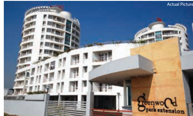
Greenwood Park Extension , Rajarhat
